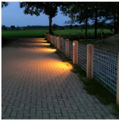
LIGHTING IN FENCE POST
